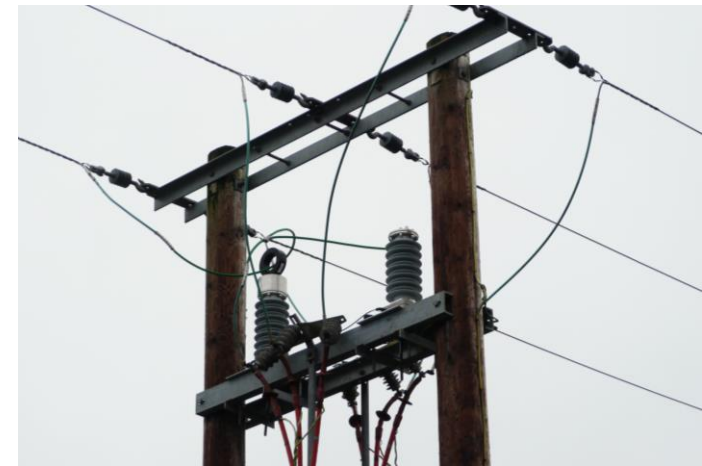
Passive Converter and CT
