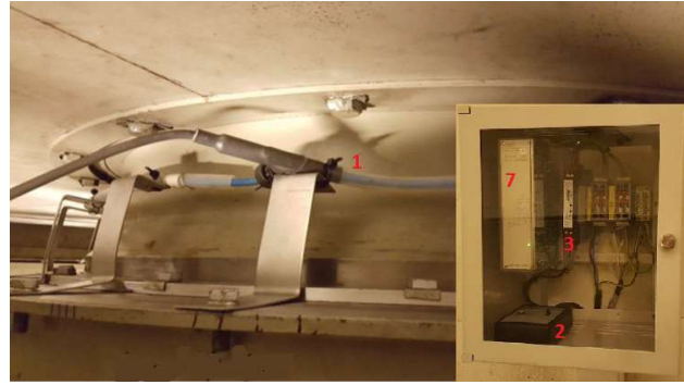
Figure 2: An actual installation of Shaft OC Protection
