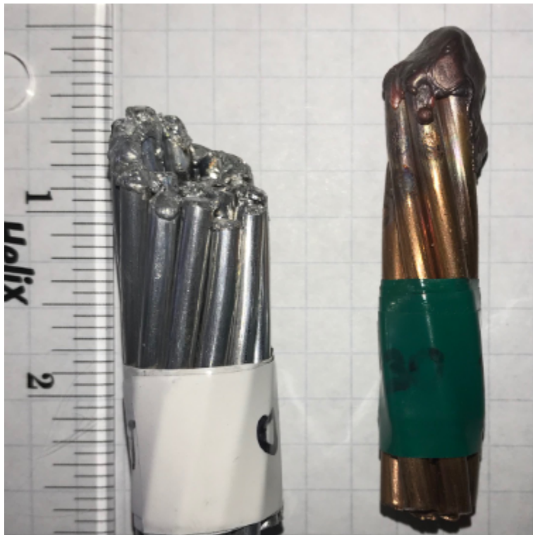
Figure 19. Comparison of typical aluminum (397 MCM Al) and copper (3/0 Cu) pigtailed conductors after fault testing. Both conductors were at approximately the same starting point prior to the test initiation.
