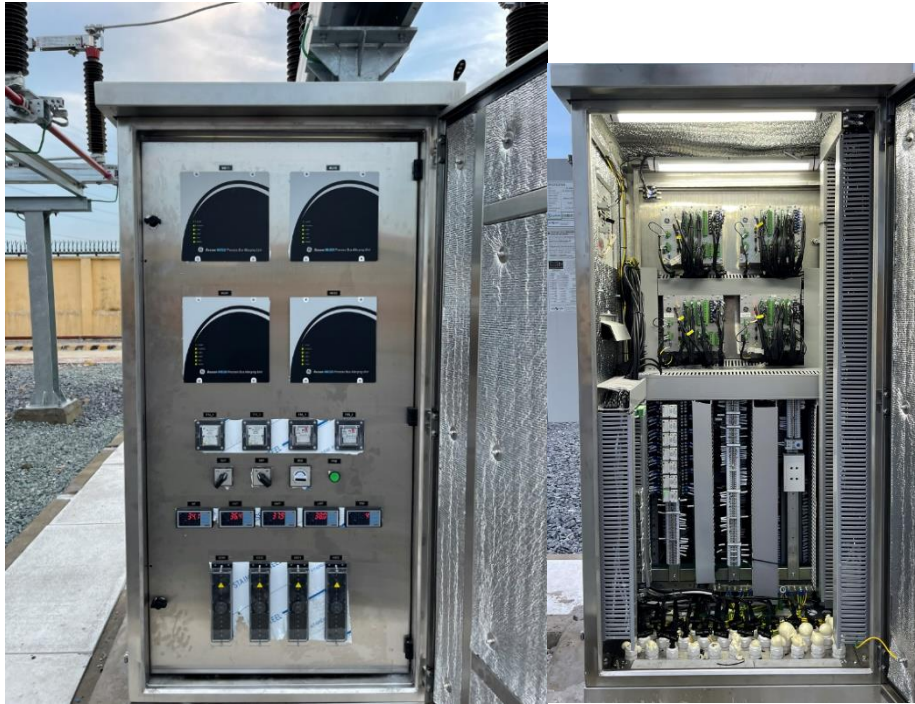
Figure 7: The MU units in the outdoor cubicle at 110KV Nghi Son
