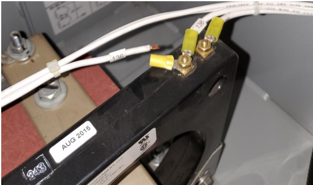
Fig 21: CT connections that came off
