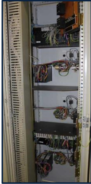
Figure 4 -Traditional Wired Relay Panel vs. Digital Substation Relay Panel
