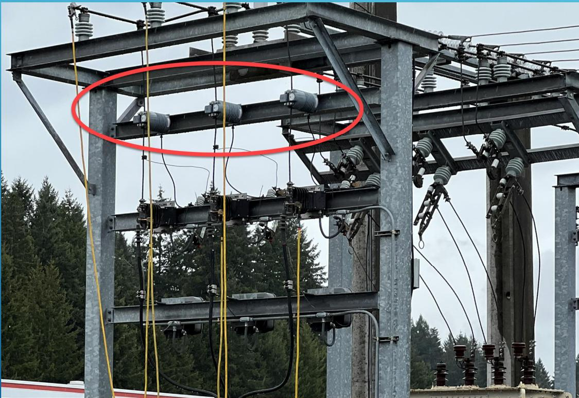
Main hurdle: the cable length from the voltage divider output can have a maximum length of 35'
