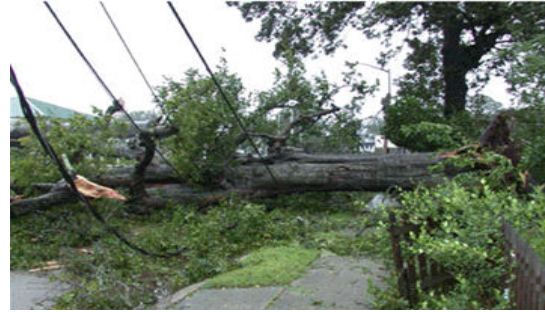
Fig. 1. Downed conductors
