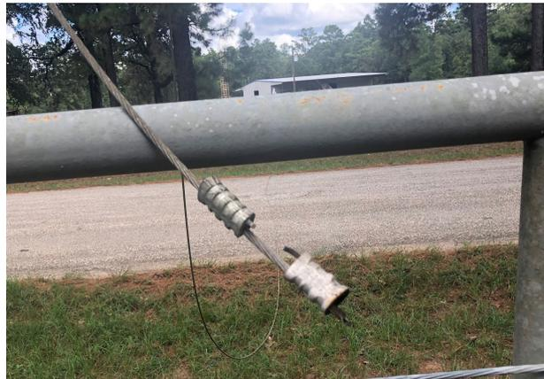
**Subject Case** – This case involved a manually operated blade switch mounted on the metal structure in a rural, unmanned 25 kV substation. The switch is shown in the photograph at right. The substation’s single power transformer had three distribution circuits, and the subject switch carried the load for one of the circuits. At the time of the incident, the switch was carrying load, and the utility company had no active customer complaints or conventional indication of a problem.
