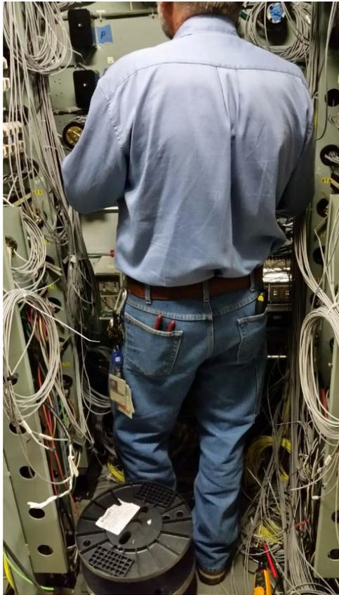
Relay cabinets are booth shaped enclosures with equipment and live terminals typically on three sides. All cabinets have doors and many have swinging equipment panels and thresholds.
